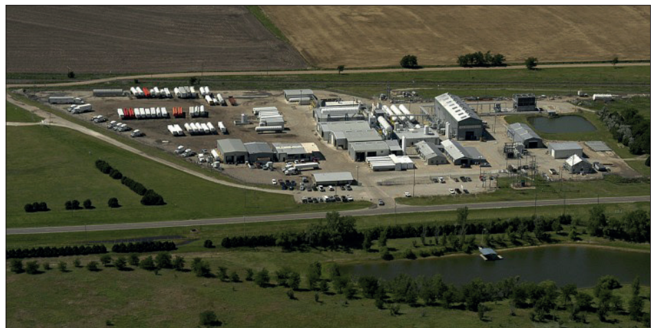
An aerial view of Linde's Otis, Kansas Helium Plant. Photo courtesy of Linde.
